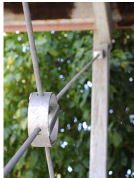
Inspect bracing on decks and balconies for undue structural movement
