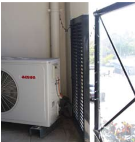
Avoid placing climbable objects close to balustrades or opening windows
